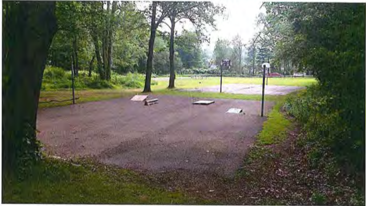
Figure 5, view of asphalt courts.
