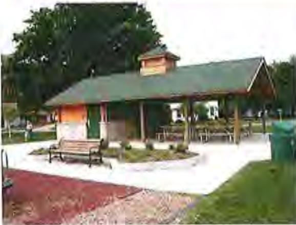
Figure 35, multi-purpose pavilion with integrated restrooms.
