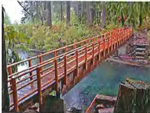
Figure 37, timber pedestrian bridge.
