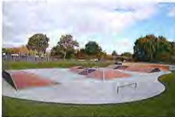
Figure 34, concrete skate park.
