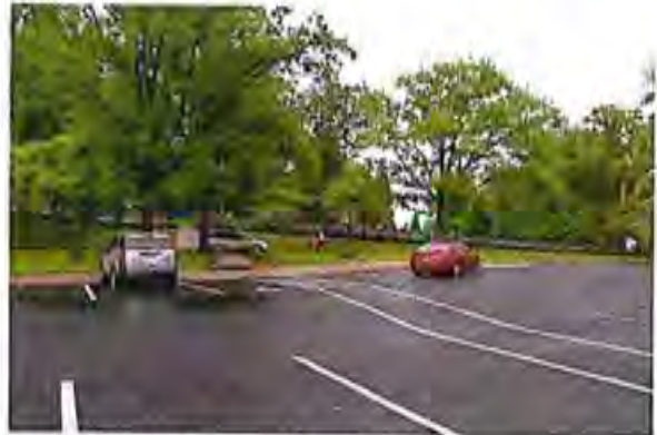
Figure 20, asphalt paved parking lot.
