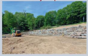
The stacked stone wall has been completed. Stormwater pipes and drainage systems are still being installed. Site work for the stairway, curbing, playground equipment and playground surface has started. The parking fencing is being installed. The contractor has brought in a top soil screener to screen excavated soils at the project into top soil for final grading and planting.
