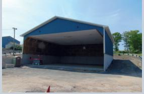
Construction of the salt shed is completed. The stormwater inlets and piping are being installed along with construction of stormwater retention pond site grading and grass seeding. Weather permitting work is scheduled to be completed by June 11th.
